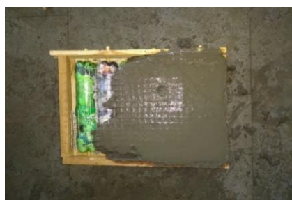
Figure 12 Plastering the upper layer of the bottle panel
