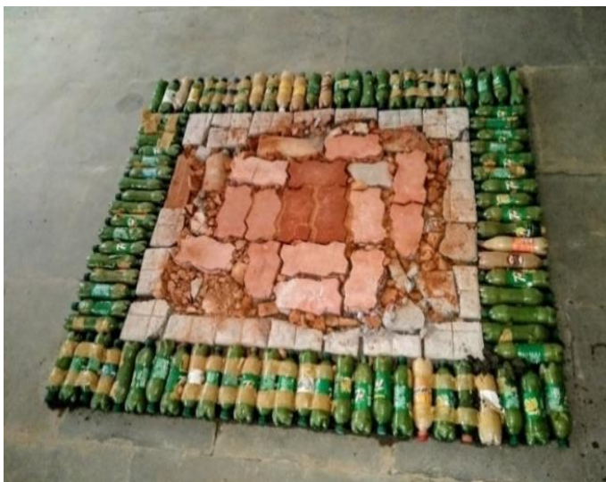
Figure 18 Construction of basement
