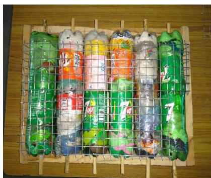
Figure 11 Bottle units placed in wooden frame and chicken wire mesh placed above
