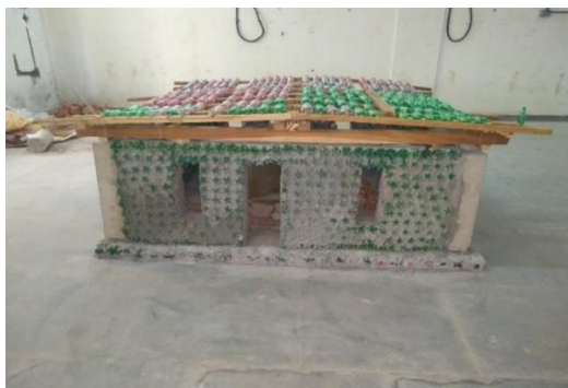
Figure 26 Roof placed above the walls
