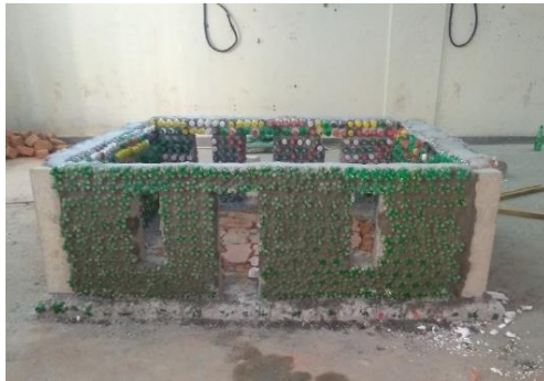
Figure 23 Completed stage of walls
