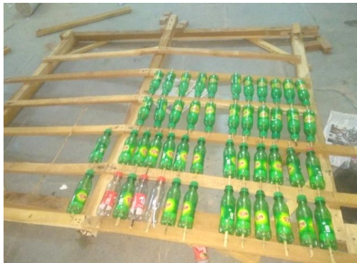
Figure 24 Construction of roof
