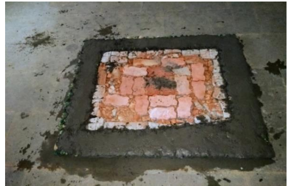
Figure 19 Completed stage of basement
