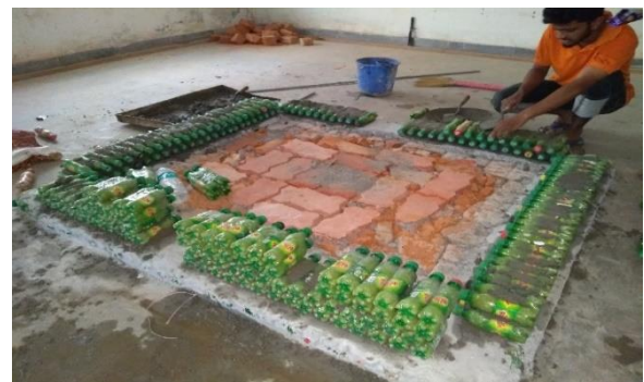
Figure 20 Construction of outer walls
