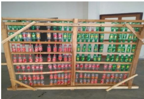
Figure 25 Completed stage of roof
